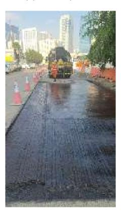
We have 02 nos pavers with all the relevant machinery comprising the set. The set includes Tandem Rollers (DDR) and Pneumatic Tiered Rollers (PTR) with Mini Rollers for making jointing as well as small patch operations where limited space forces to use small equipment.
